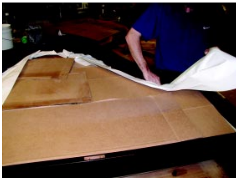
Photo 5 — Once the soundboard and plate are covered with cardboard, tape a 15 in. width of paper around the perimeter.
